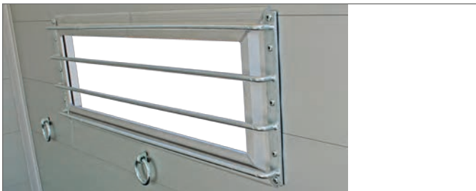
Bars (interior view)
