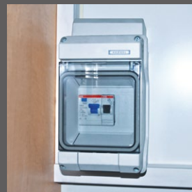
Distribution box with RCD and fuse (16 A)
