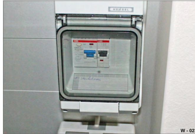
Fig. 23 Inside power distributor box
